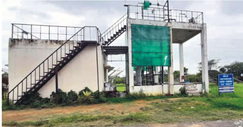
Figure 4.6 Solar water pump test facility for up to 10 hp
