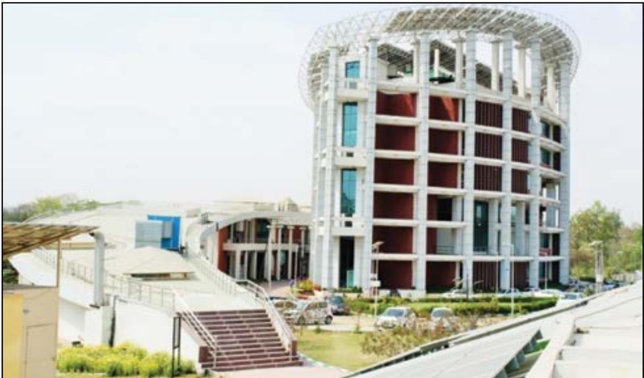
Figure 2.2: Surya Bhawan Building of NISE
