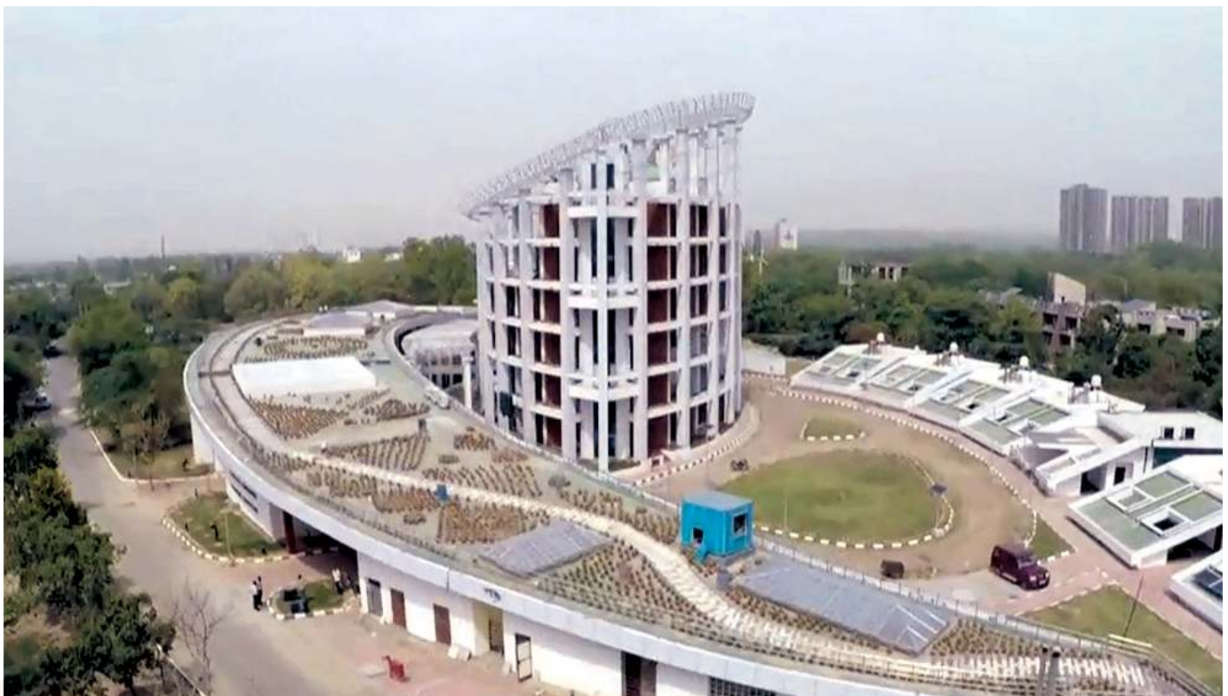
Figure 1.2: Surya Bhawan Building of NISE
