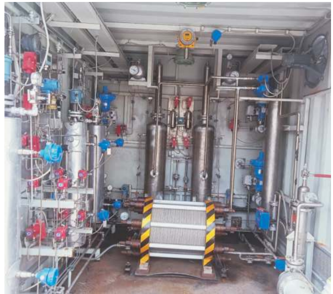
Figure 2.11: Installation of new electrolyser at NISE hydrogen generation facility
