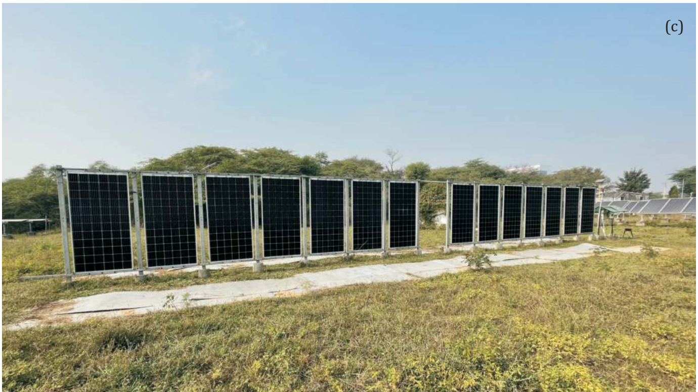
Figure 2.4: Photograph of the Solar PV power plant (a) Mono facial at latitude tilt (10 kWp), (b) Bifacial at latitude tilt (5 kWp) and (c) Bifacial at vertical tilt (5 kWp).
