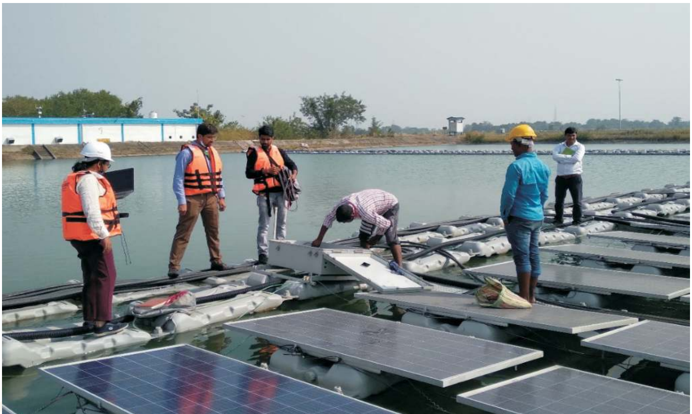
Figure 5.1: On-site performance mapping of floating SPV (WBPDCL, West Bengal)
