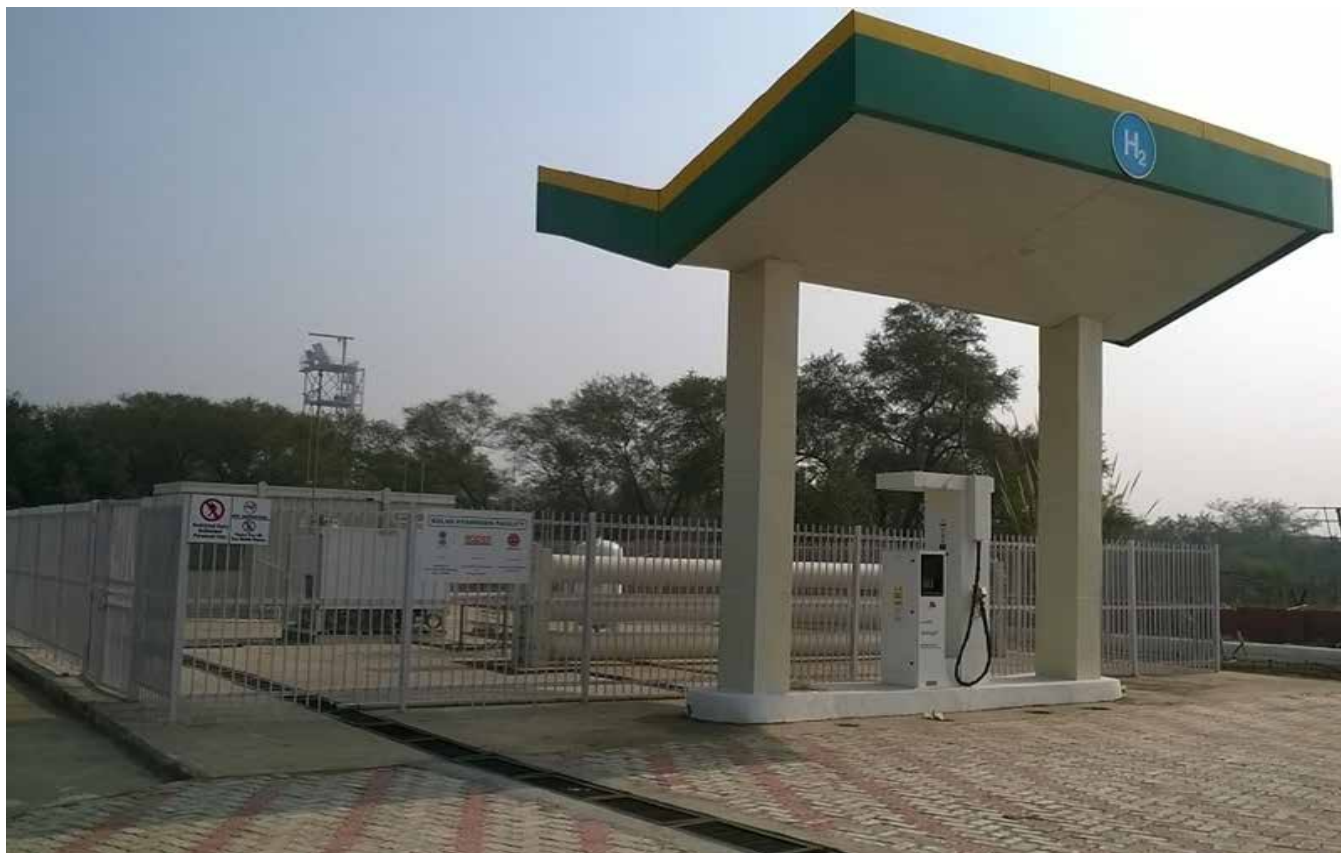
Hydrogen Refuelling station at NISE, Gwal Pahari
