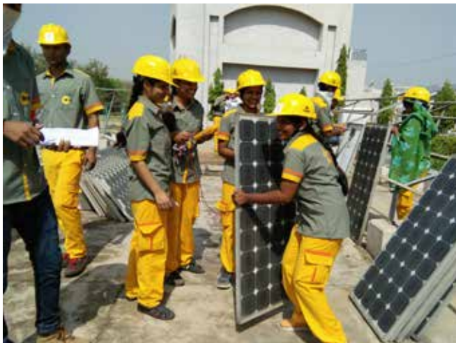
Work at site, NISE Haryana
