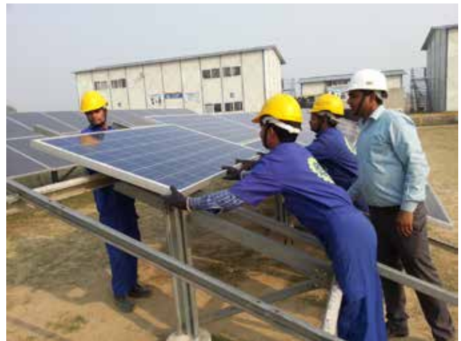
Work at site, L&T, Pilukhwa, UP
