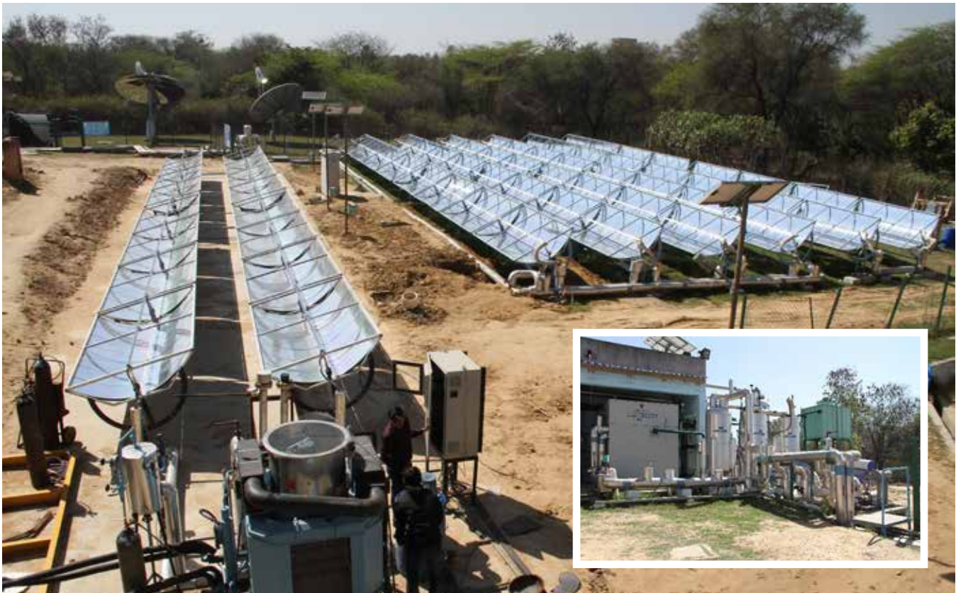
100 kW High Efficiency Triple Effect Vapor Absorption System
