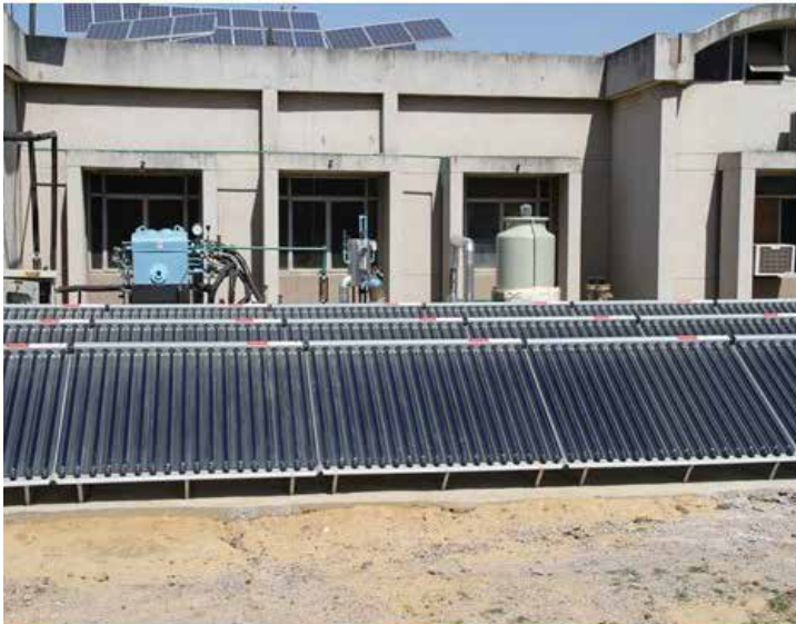
Figure 5.7: 5 kW Adsorption Refrigeration system
