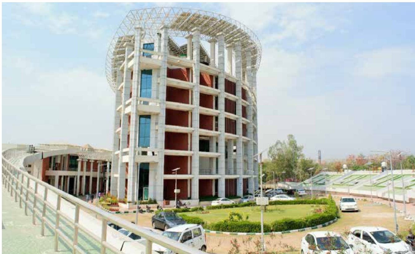
Figure 2.1 : Surya Bhawan Building at NISE, Gurugram
