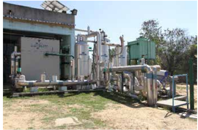
Figure 5.5: 100 kW High Efficiency Triple Effect Vapor Absorption System
