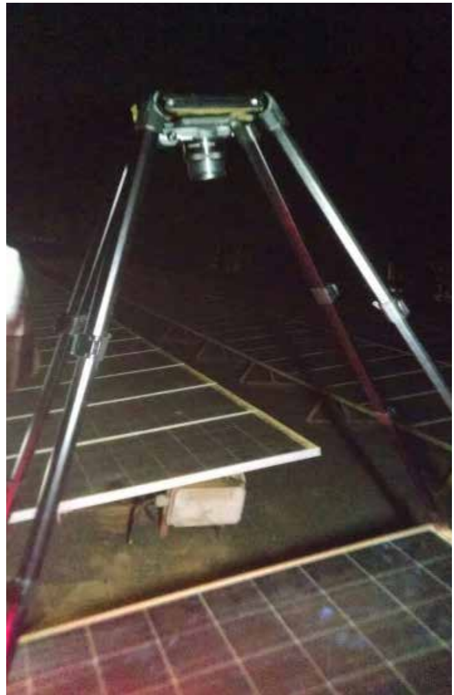
Figure 10.1 : EL Testing performed at power plant site
