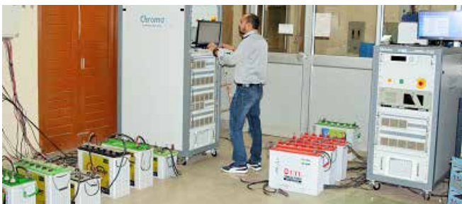
Figure 4.4: Test set up of battery testing laboratory
