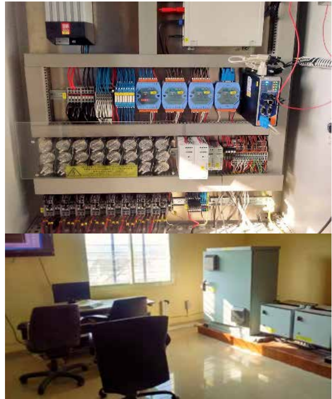
Figure 4.17: Test set up for IV tracing of PV Module
