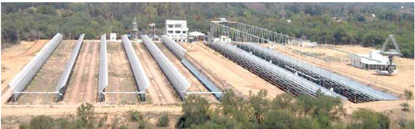
Figure 5.1: PTC and LFR Solar fields of the 1MWe STPP at NISE
