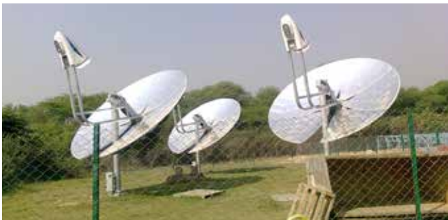
Figure 5.5: Solar Dish Stirling System
