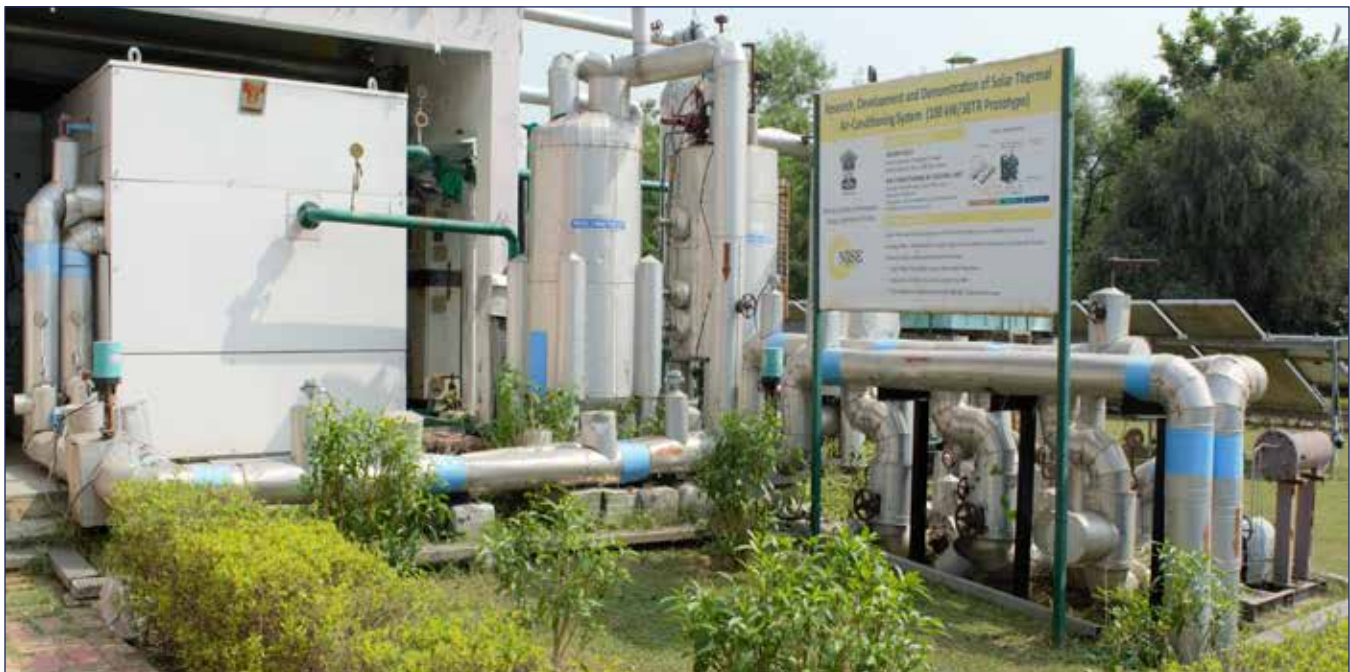
Figure 5.2: 100 kW triple effect vapour absorption system
