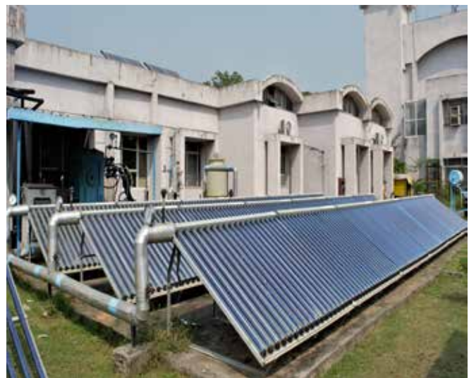
Figure 5.4: 5 kW solid Vapour Adsorption System
