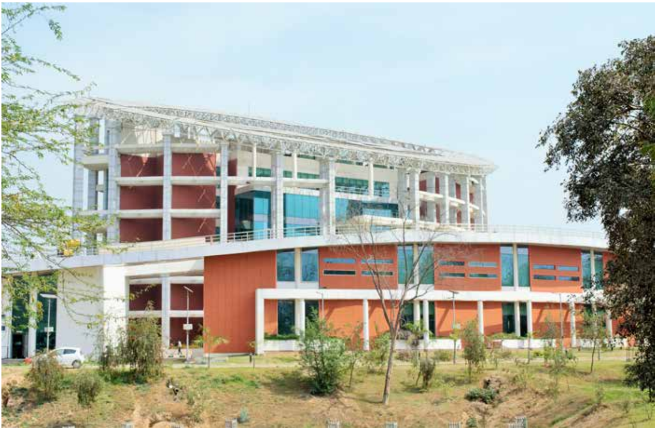
Figure 2.1: Surya Bhawan Building at NISE, Gurugram
