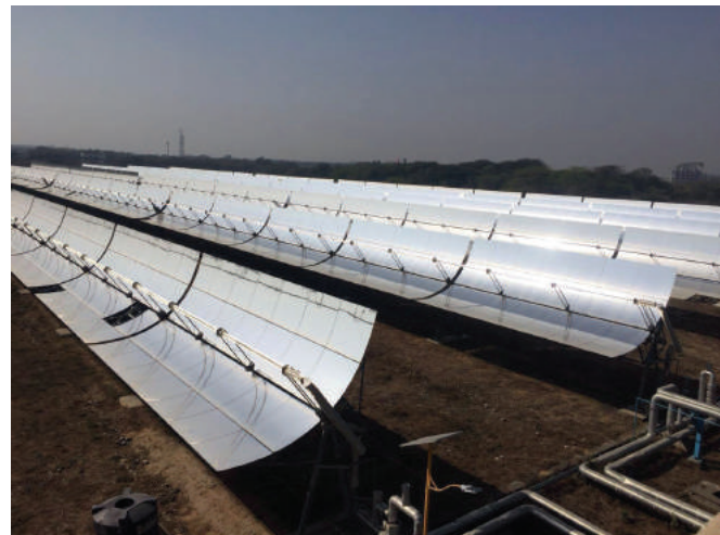
Figure 5.4 PTC Solar fields of the 1.0 MWe STPP at NISE
