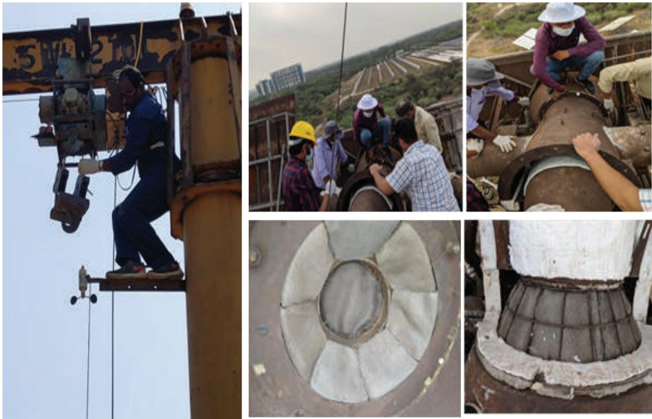
Figure. 7.21. Various O&M activities at Modular Central Receiver Power Plant
