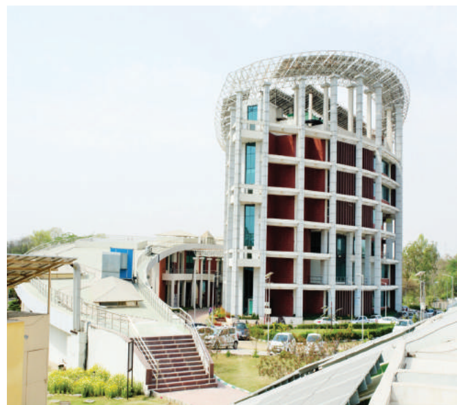
Figure 2.2. Surya Bhawan Building at NISE, Gurugram
