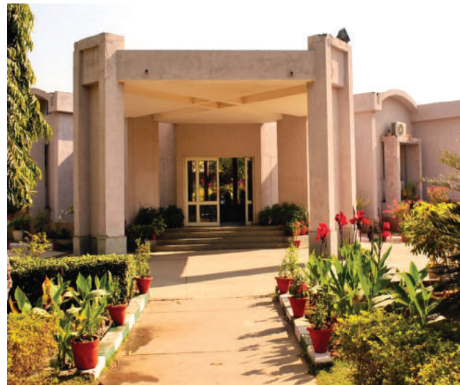
Figure 2.1. Aditya Bhawan Building at NISE, Gurugram
