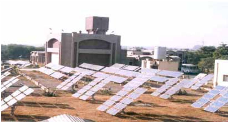
25 kWp crystalline silicon module test bed
