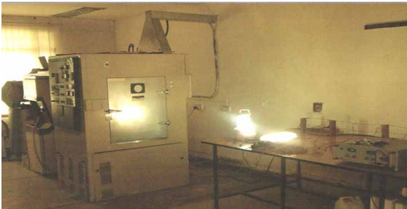
PV lighting system testing and evaluation facility
