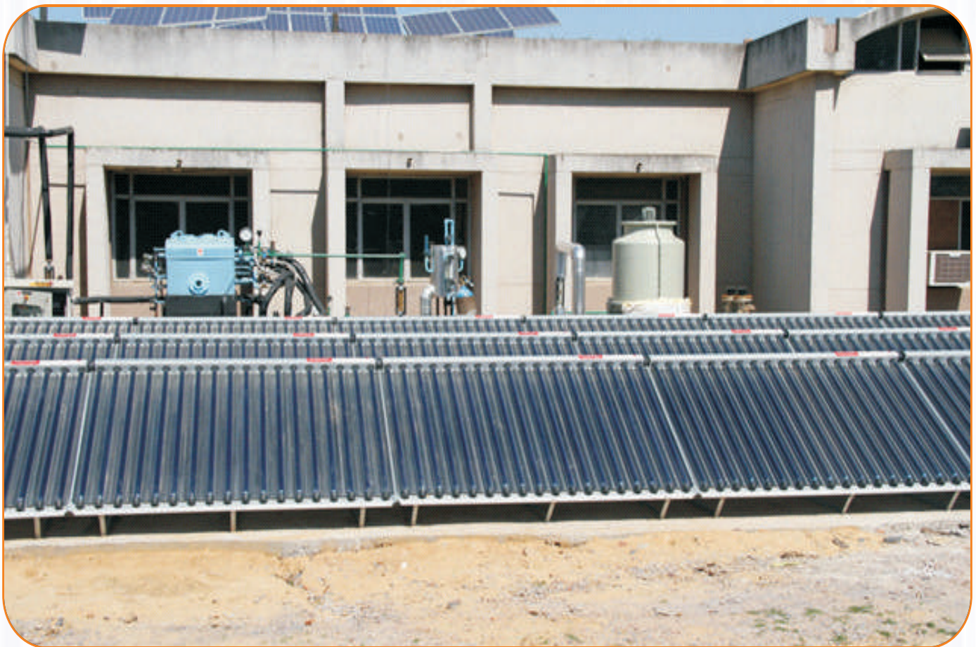
Fig. 3.7: 5 kW Adsorption Refrigeration system
