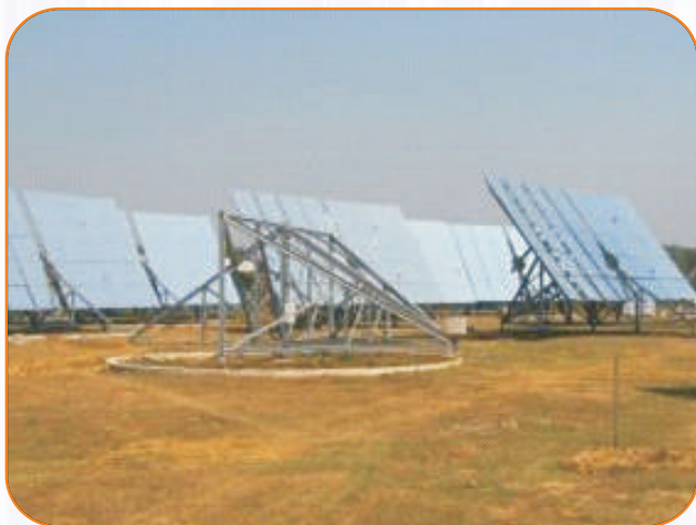
Fig. 3.3: Central Receiver Solar Power Plant
