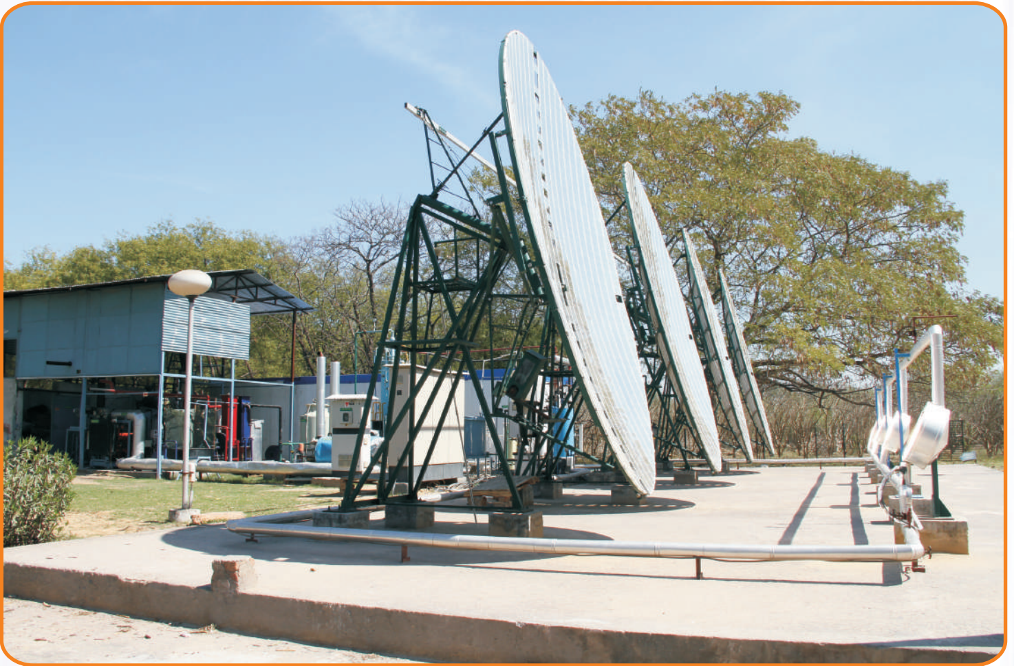
Fig.3.9: Solar Biomass Hybrid Cold Storage System
