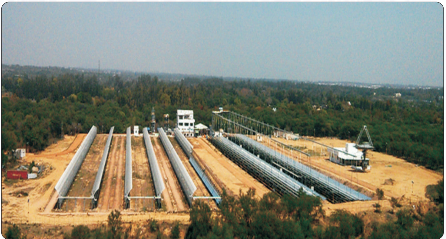
Fig. 3.1:1 MW Solar Thermal Power Plant at National Institute of Solar Energy
