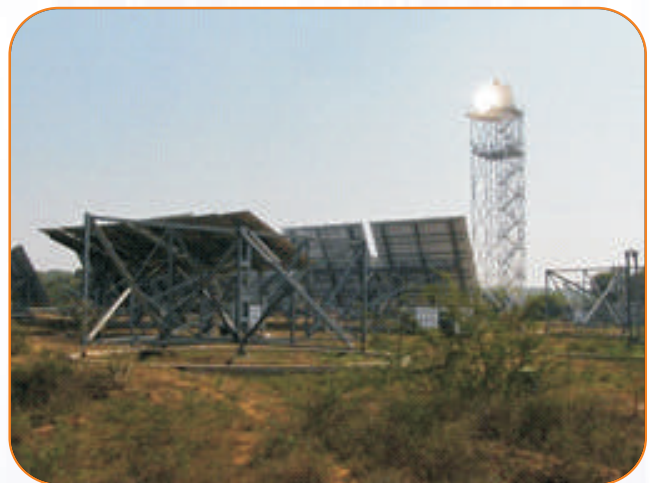
Fig. 3.3: Central Receiver Solar Power Plant
