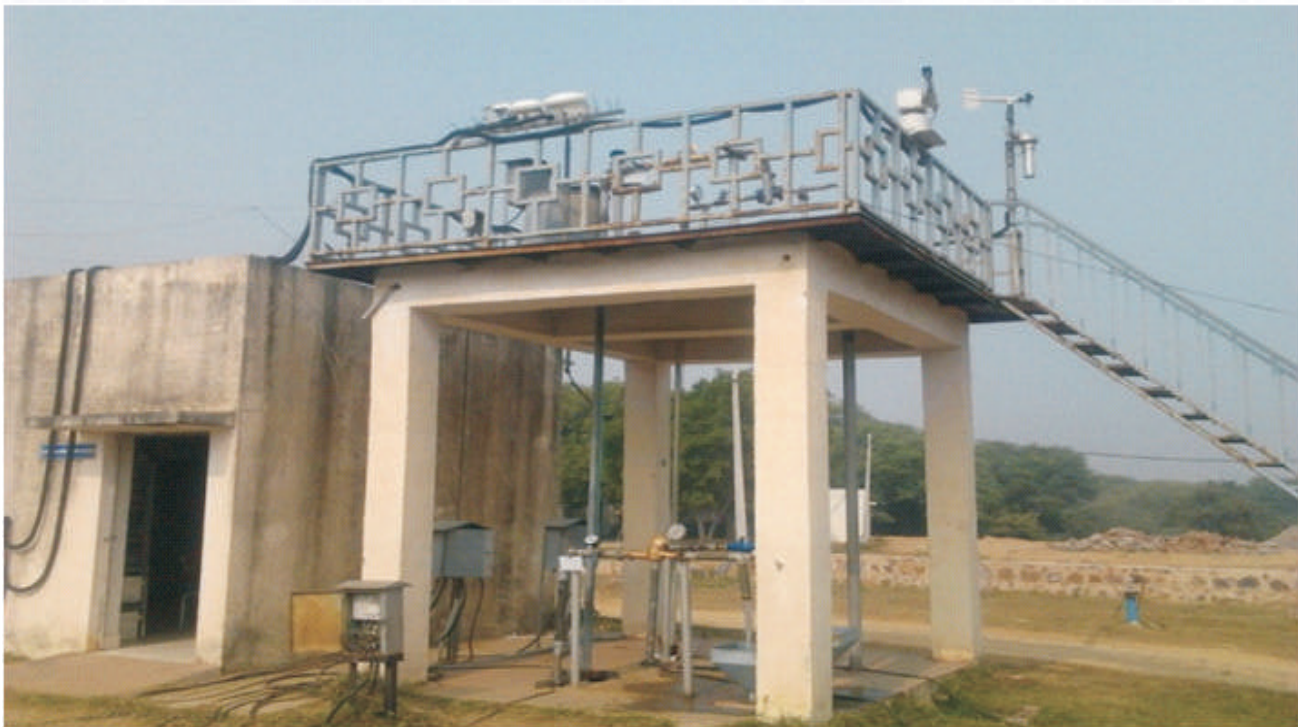
Solar Water pump test Facility
