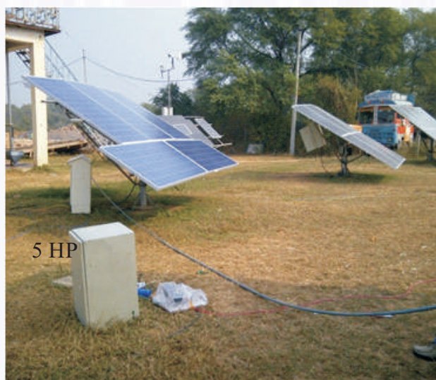
SPV module setup for pump testing at test bed
