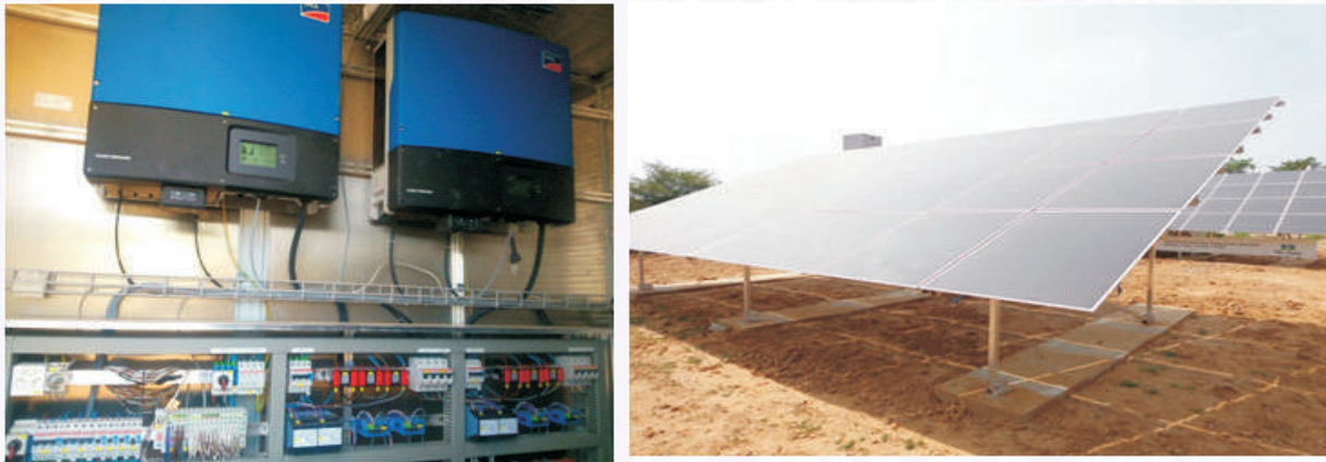
Fig. 6 Micro-morph based thin film PV technology test bed at NISE
